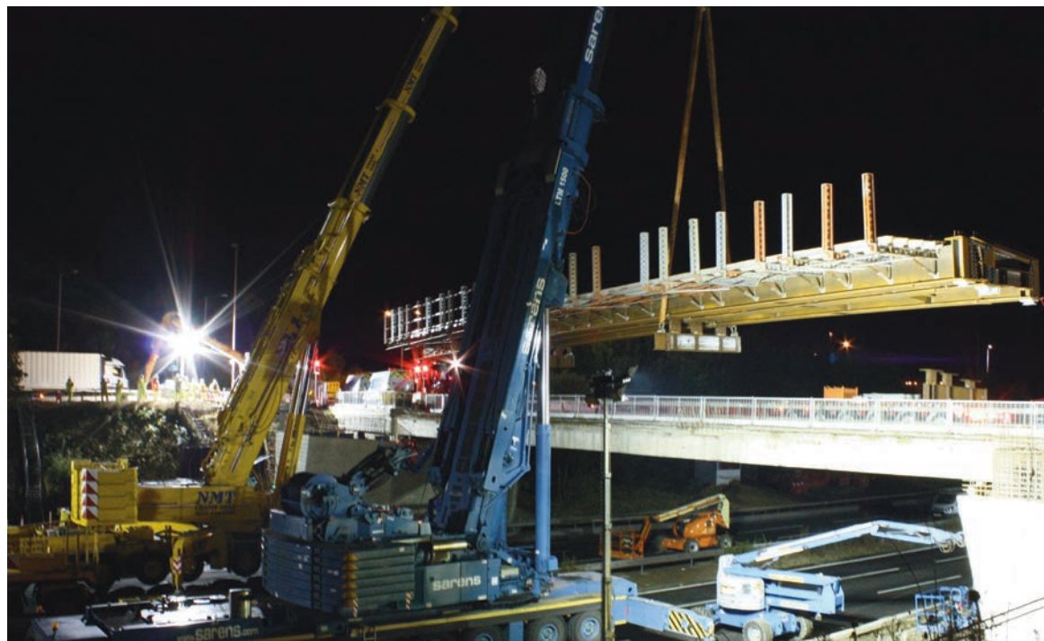
M20 Junction 4 overbridge widening
